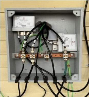
VE7PTN home station antenna coax junction box (cover removed) showing temporary installation of LNA external preamplifiers and mode J filter (on LNA on right side)
