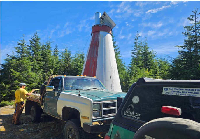
The Woss Repeater site
