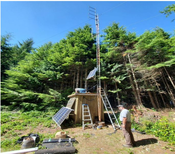
Work at the Shelly Mountain site
